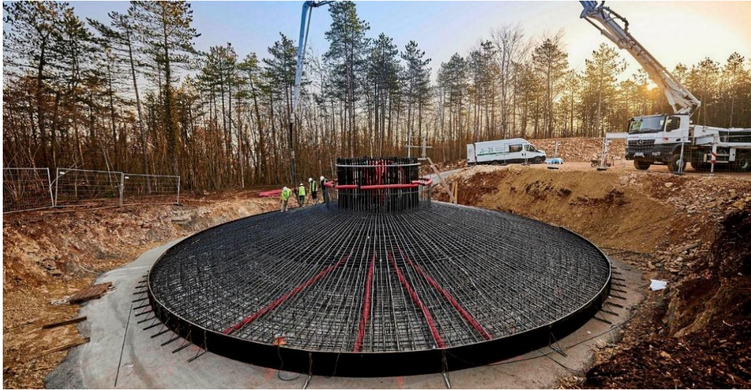
Figure 2.11. Wind turbine foundation.
