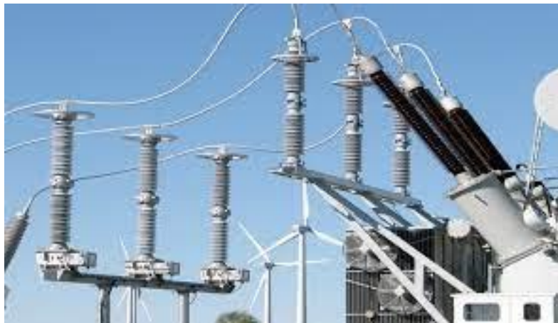
Figure 2.6. Lightning Arrester.
