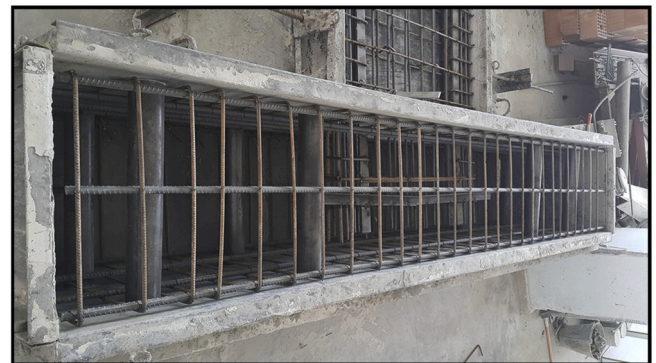
(b) Elevation view of foundation reinforcement.
