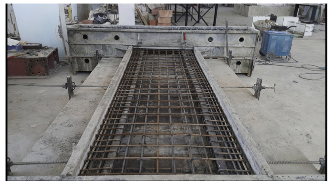
(a) Elevation view of shear wall reinforcement.
