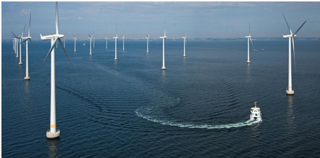
Figure 2.9. Offshore wind farm (Øresund between Malmö and Copenhagen, Sweden)
