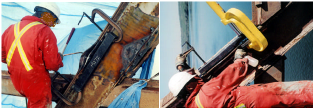
Figure 2.3. Heat treatment of steel girders [7].
