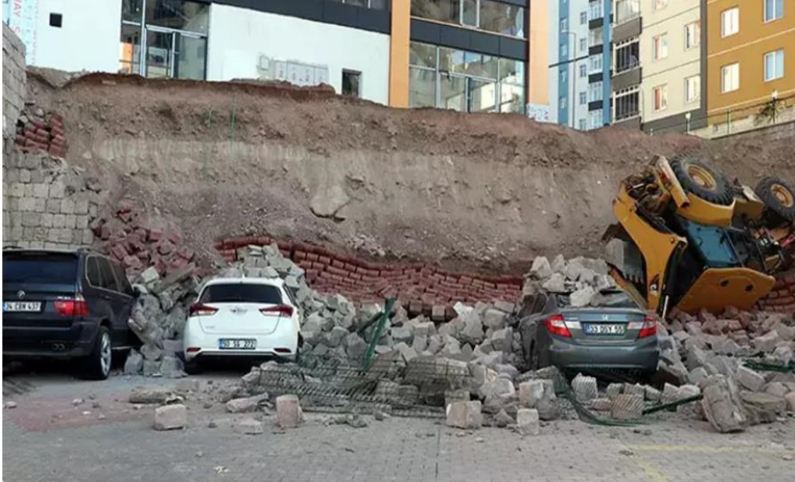
Figure 2.9. Collapsed example of retaining wall in Kayseri (url2, 2021; Sönmez, 2023).
