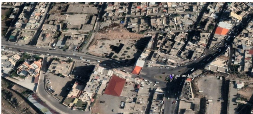
Figure 3.6. Close up of Rasheed junction
